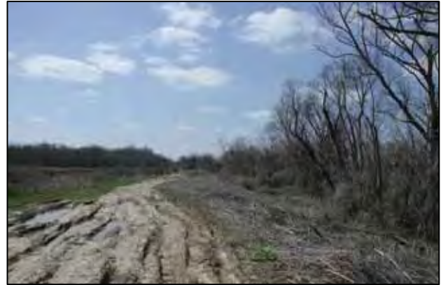
FIGURE H2. Both sides of location H had large levees used as roadbeds parallel to the river channel, bisecting the transects.
